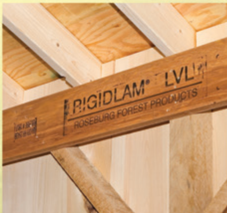
Glue LAM LVL Header for Increased Snow Loads and for Hurricane Regions
